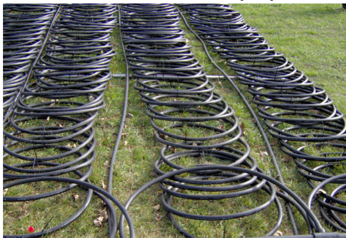
Heat pump array prior to installation
