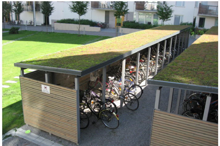
Green roof on cycle storage within a secure courtyard
