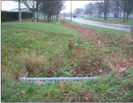
Figure 17: A dry swale (Source: SUDSnet TM )
